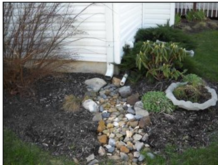
3. Downspout in rear
